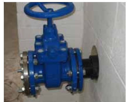
Folding flange allows easy Connection to internal pipework
