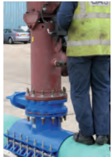
Demonstration of drilling a gas main under-pressure. The Series 214 tee is clearly visible at the bottom of the picture.
