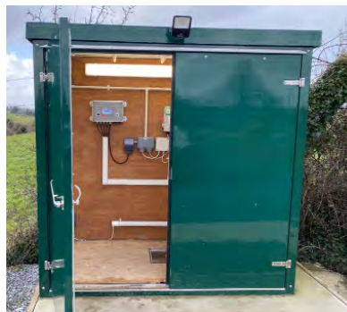
Pictured above, is the kiosk containing needle valve, actuator and controller (PMD) and the data display monitor, pictured below
