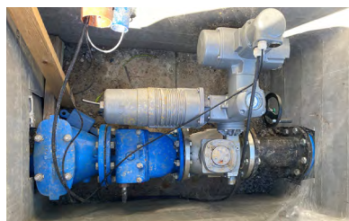
Pictured above, is the kiosk containing needle valve, actuator and controller (PMD) and the data display monitor, pictured below
