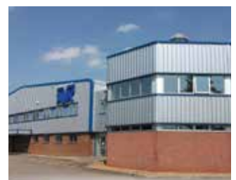
AVK Aqua-Gas Manufacturing, Corby, Northamptonshire
