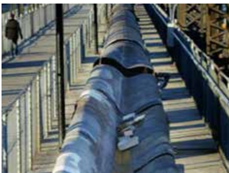
*Example of a pipeline collapse.
