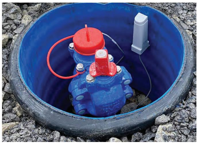
Hydrant with VIDI Temperature installed. VIDI Temperature is typically installed in combination with a gate valve, hydrant or similar. After installation, the device transmits information about the temperature in the network to the VIDI Cloud platform that stores the data.
