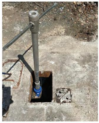
A VIDI Positioner installed in-situ underground.
