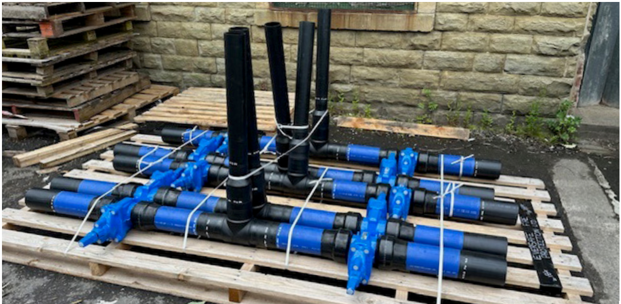
The valve fabrications were completed offsite, palletised and delivered to site
